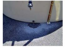
chemical tank is leaking and the dried liquid is leaving a residue on the pavement. Stuff like this happens at nearly every site. Having an active maintenance program and staying on top of little problems like this can prevent much bigger
